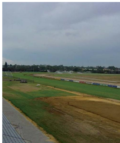
(below) Stages of the renovation of the Ascot track
